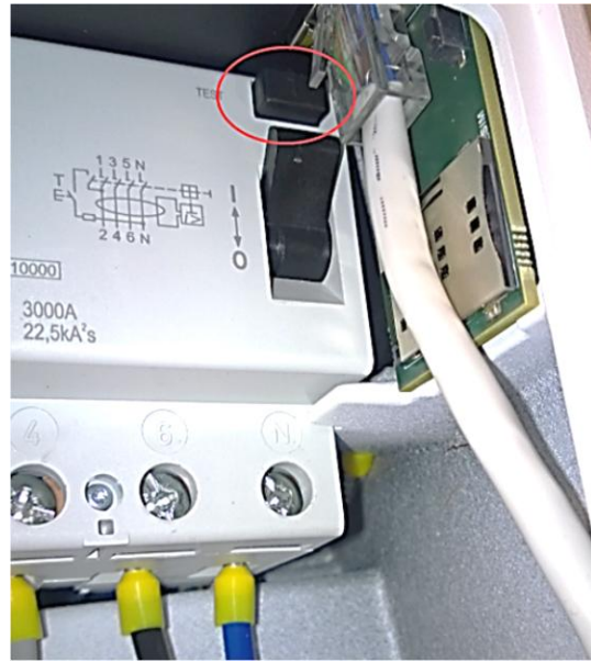
Figure 41: Bouton de test RCD
